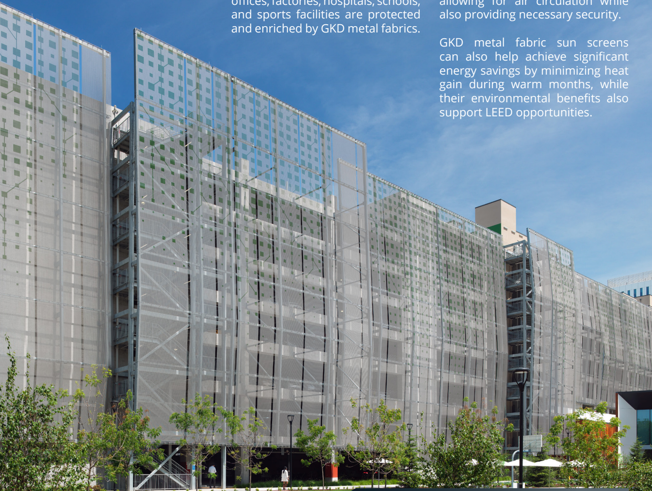
Samsung Headquarters Parking Garage | NBBJ | San Jose, CA | Omega 1520 | Woven-in-bar with Hooks & Woven-in-bar with Eyebolts attachments
