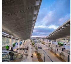
Between 2018 and the project's completion in 2024, GKD produced approximately 1,400 unique panels. Each one was individually sized and shaped to create flowing, organic forms. The fabrication process had to meet stringent LA certification requirements. Each panel was carefully crated and shipped in phases over the multi-year construction period.
